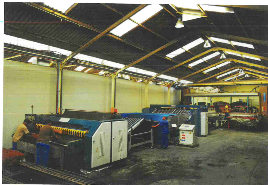
The brand new installed automated drying line from sams/setting to vacuum drying, one of the many technological improvements contributing to the tannery's strategic goals for expansion into the global market.
